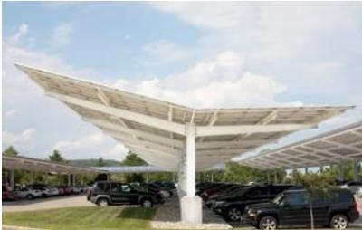
Directs snow & ice safely to the center of our patented dual-tilt canopies to melt safely away from vehicles and foot traffic
