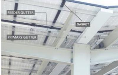
Manages storm water runoff on the underside of the canopy, while providing the potential for re-use in onsite irrigation
